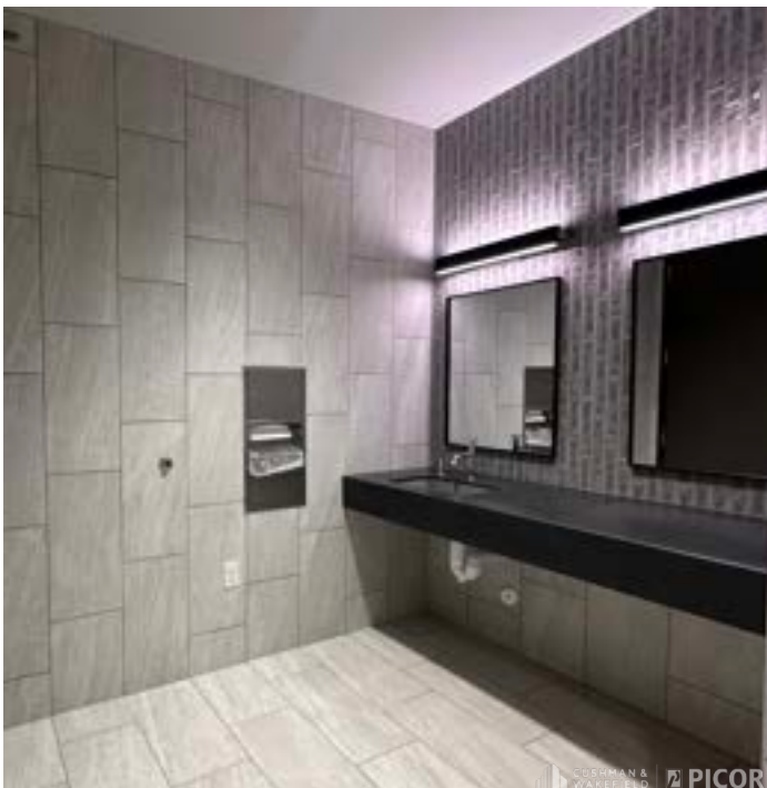
Fitness Center: New Restrooms & Showers
