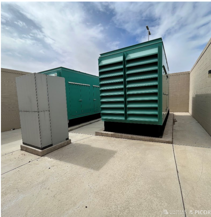
Generators – Redundant Auto-Transfer System
