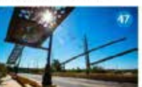
Luis G. Gutierrez Bridge, 2012 Cochise Street Artist: Brenda Geronik and Structural Quasi Inc. ARCHIT: Dean Cooper
